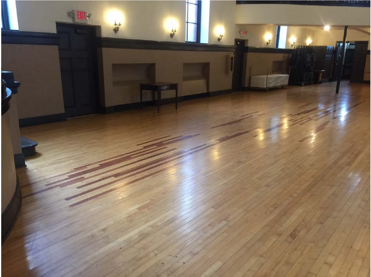
C. Main Floor, Front Right (Firehouse Side) (approximately 232 linear feet)
