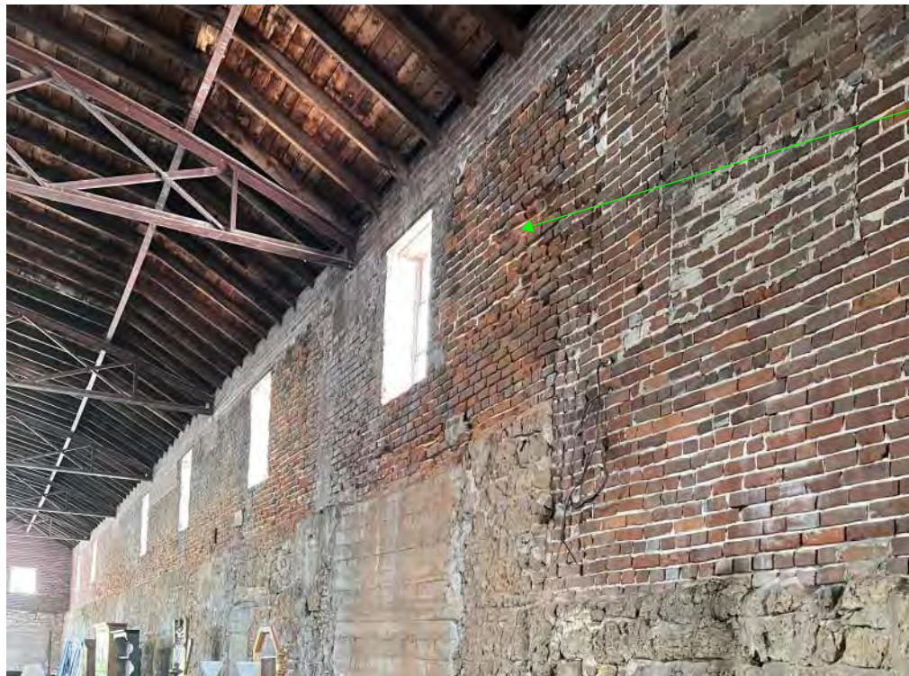
INTERIOR CONDITION OF WEST WALL
