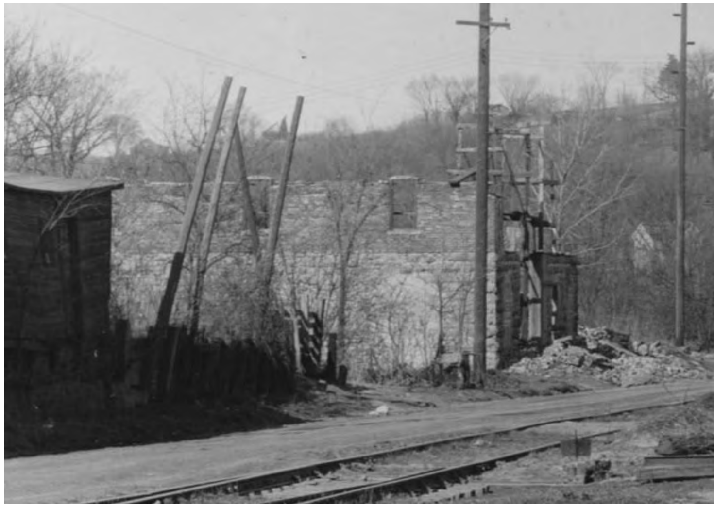
SNIP OF PHOTO TAKEN ON 2 APRIL 1946 - LOOKING EAST, REMAINDER OF WEST AND SOUTH WALLS VISIBLE
